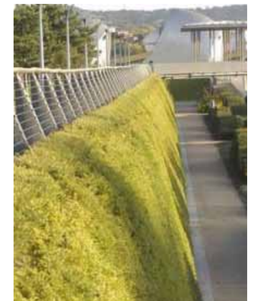
Thames Barrier Park, London, UK
